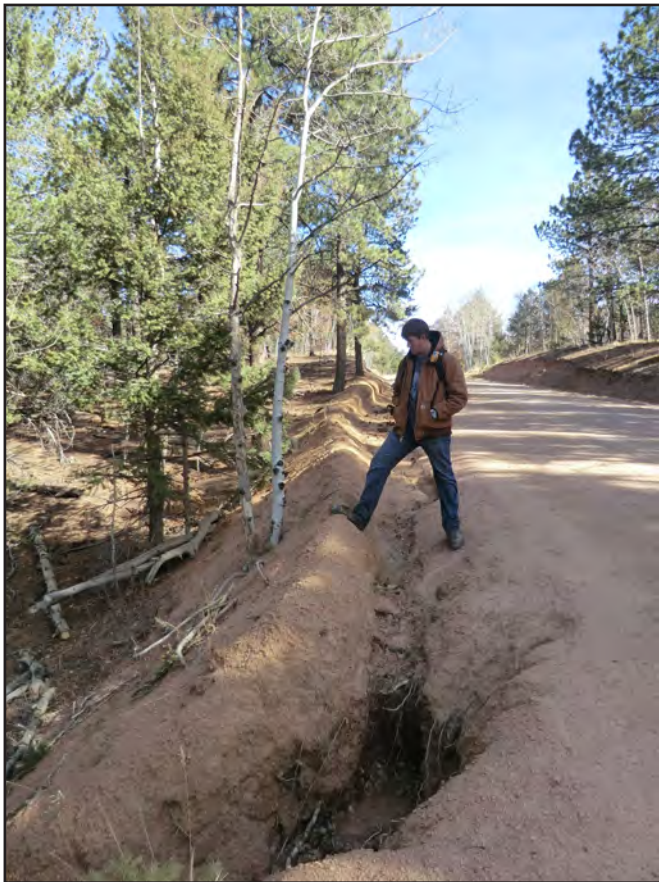
Figure 25. Road ditch with berm delivering sediment into stream channel.
