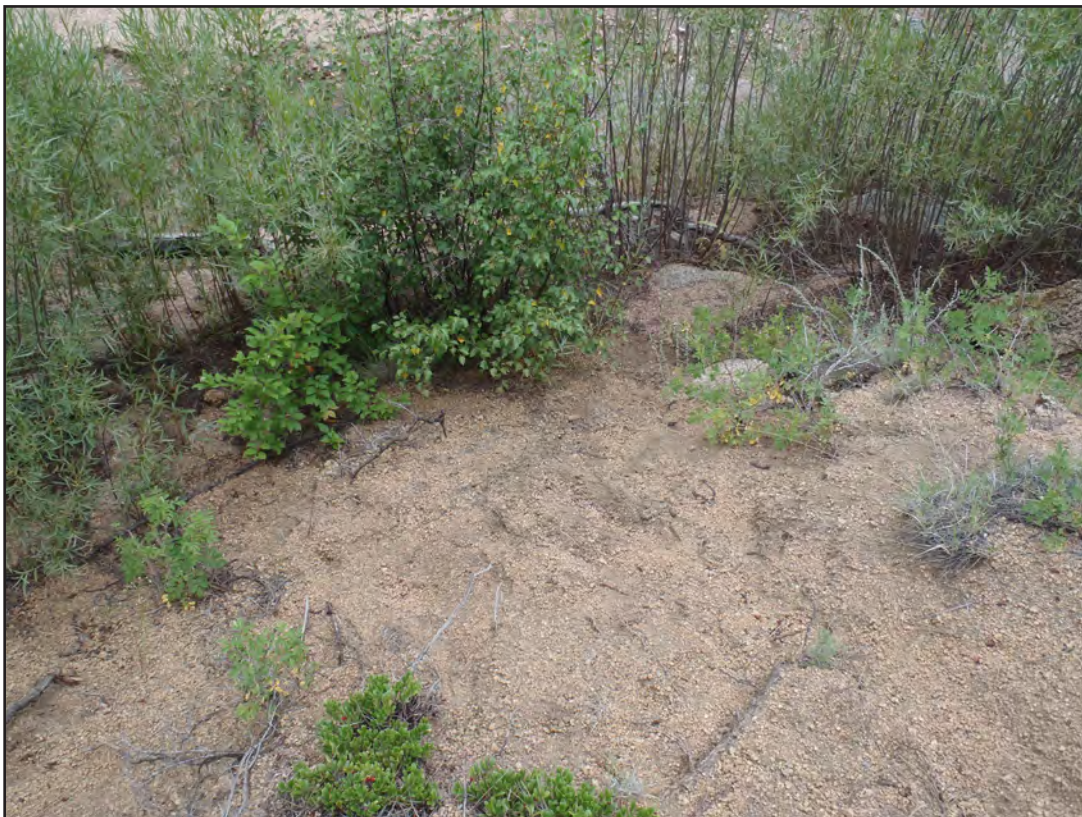
Figure 21. Close-up view of the effectiveness of the bankfull bench and riparian vegetation at preventing soil from entering stream.
