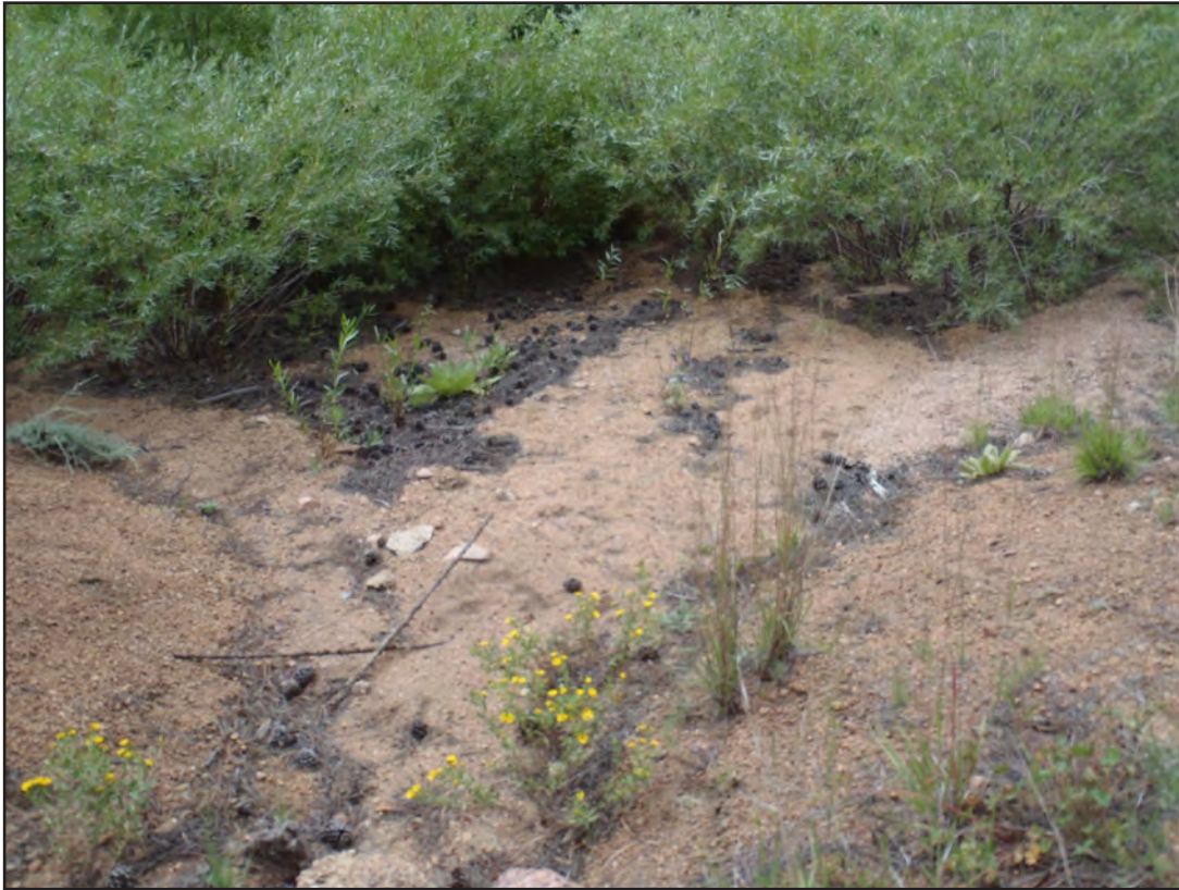
Figure 27. Small alluvial fan deposit showing stable, functioning fan and a D4 stream type at the toe of a slope as the deposit is spread onto floodplain surface preventing direct introduction of sediment.
