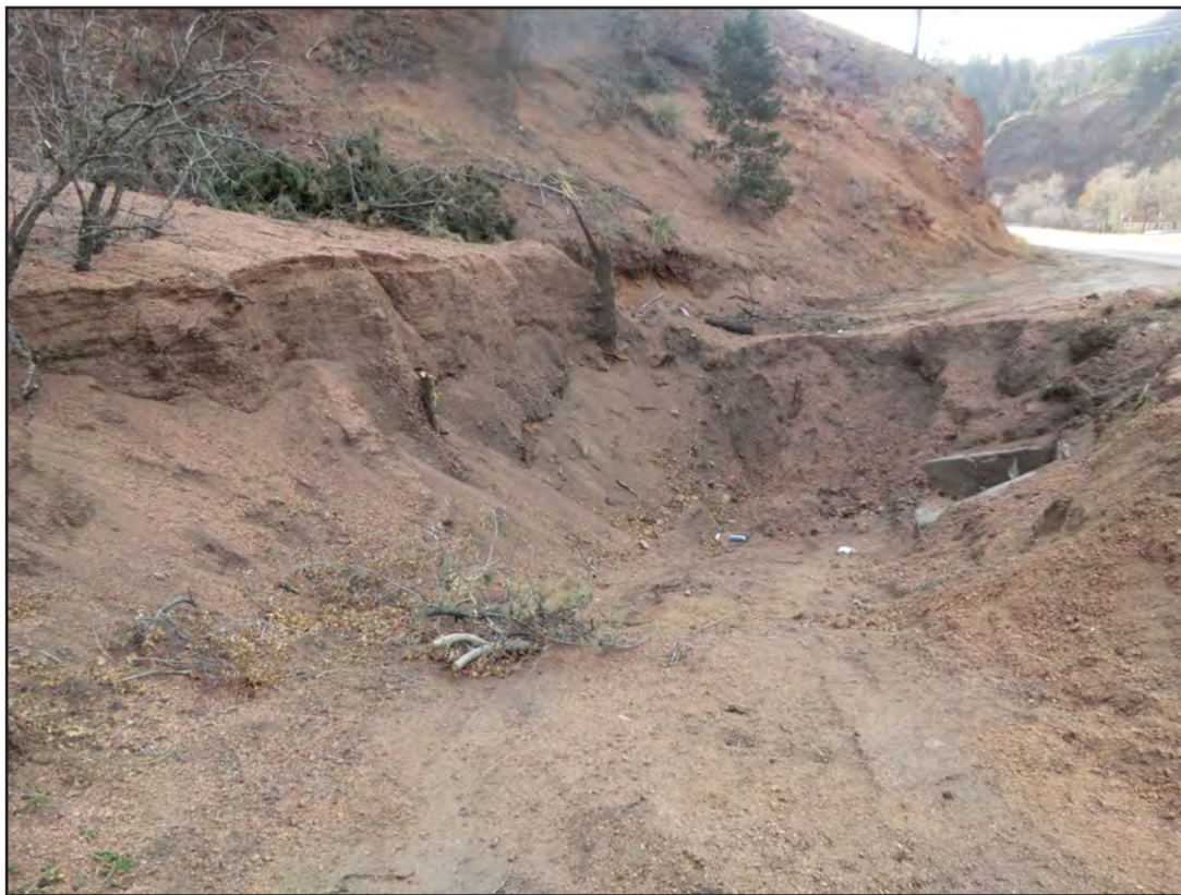
Figure 23. Cleaning out drainage structures continues to cut through depositional surfaces and cause headcut migration.
