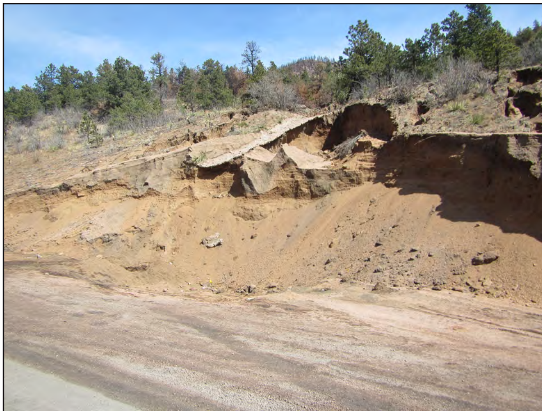
Figure 24. Road with a cut off fan accelerating erosion.
